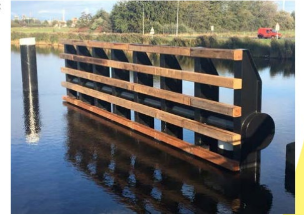
Guiding structure near Heemkes bridge
