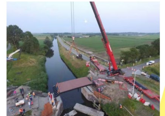
Installation of the bridge deck of re-used composite
