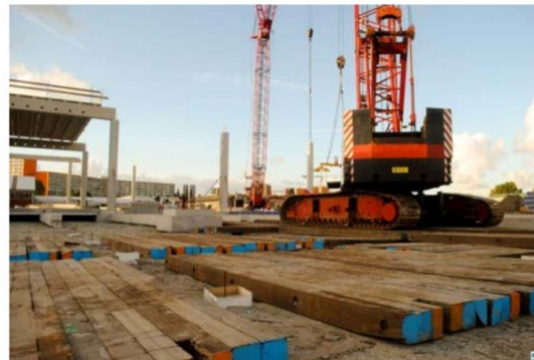
Crane mats of Welex applied at a building site
