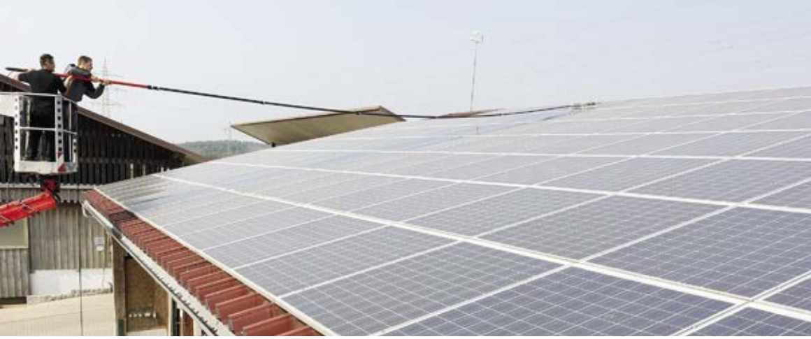
Photo: Exel Composites Oyj Photo on previous page: Ekin Muovi Oy
