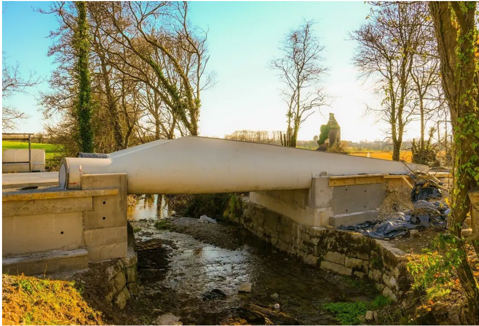
Two discarded turbine blades were used to construct the bridge outside Cork City. From: Bloomberg
