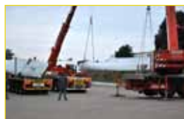
Fig.1 : Unloading of windmill blades at processing site Courtesy: Zajons, Melbeck
