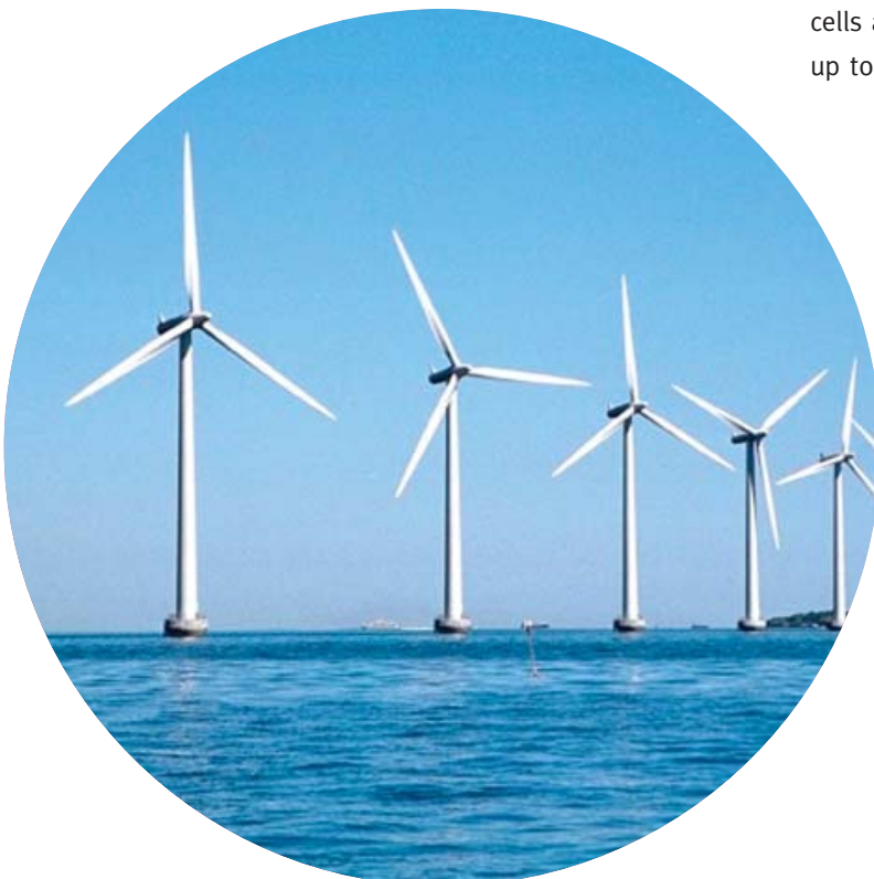
Modern wind turbines are made using fibre-reinforced plastics, thereby reaching wingspans of up to 60 metres.
