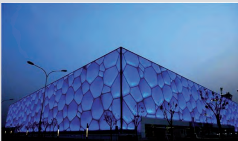
Figure 13. Innovative applications in construction: the exterior of the Beijing National Aquatics Centre, the world's largest building covered entirely by ETFE (ethylene tetrafluoroethylene)
