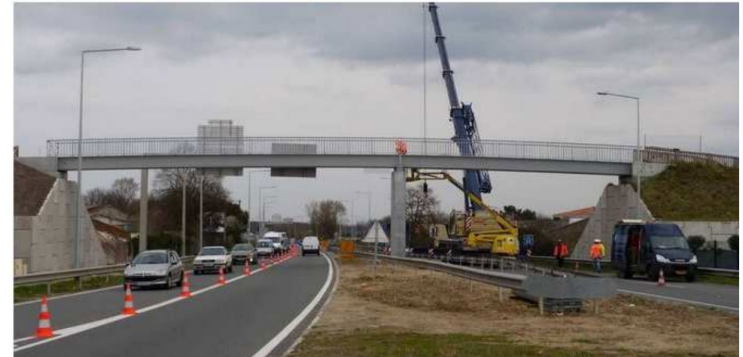
Figure 1. Pedestrian FRP Bridge, Saint-André de Cubzac, France, ©Photo P. Charbonneau
